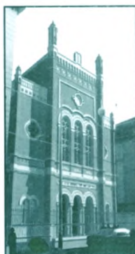
The Zagreb synagogue (destroyed 1941)
