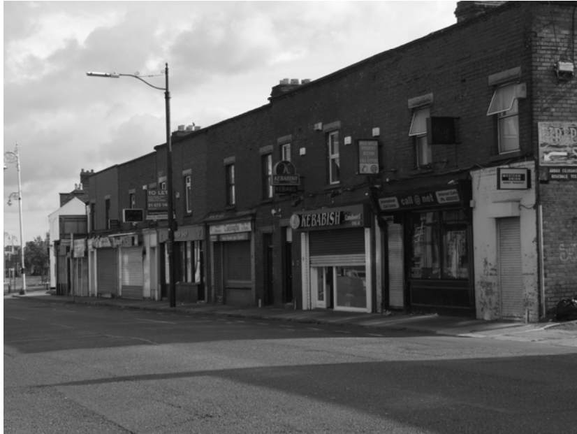
Fig. 2(xv) A terrace of small shops on Clanbrassil St., Dublin, all of which were formerly kosher shops servicing the local Jewish community until the 1980s.
