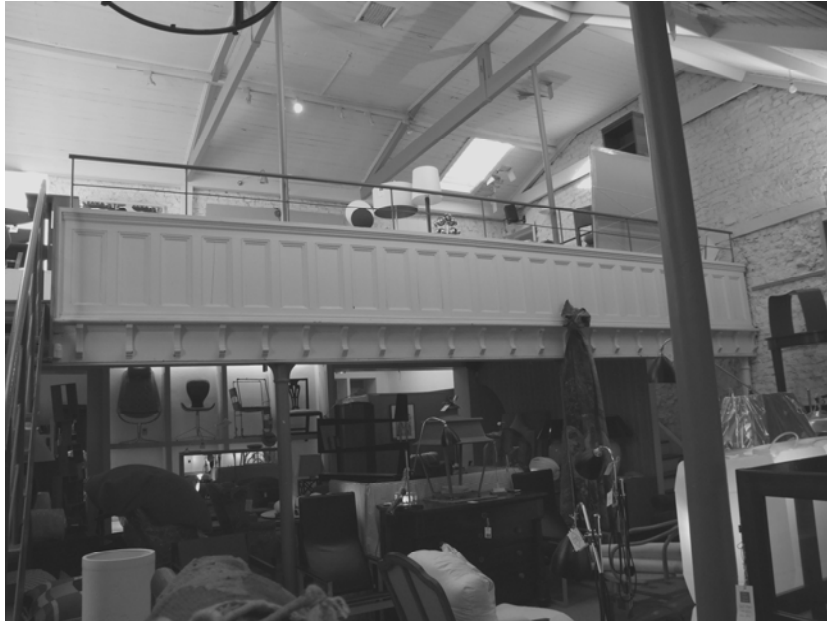
Fig. 3(vii) A view of the women's gallery in the former Lombard St West synagogue, now a furniture showroom. Note the chain-mail mechitzah has been replaced with an iron railing. (Photograph: M. Brown, 15/11/10).
