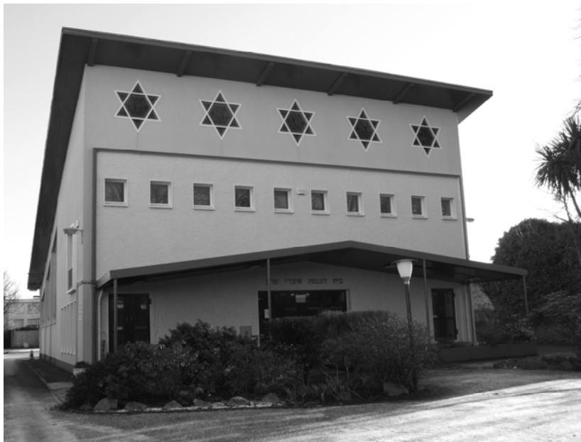
Fig. 3(iv) Exterior view of Terenure synagogue. (Photograph: M. Brown, 05/01/10).
