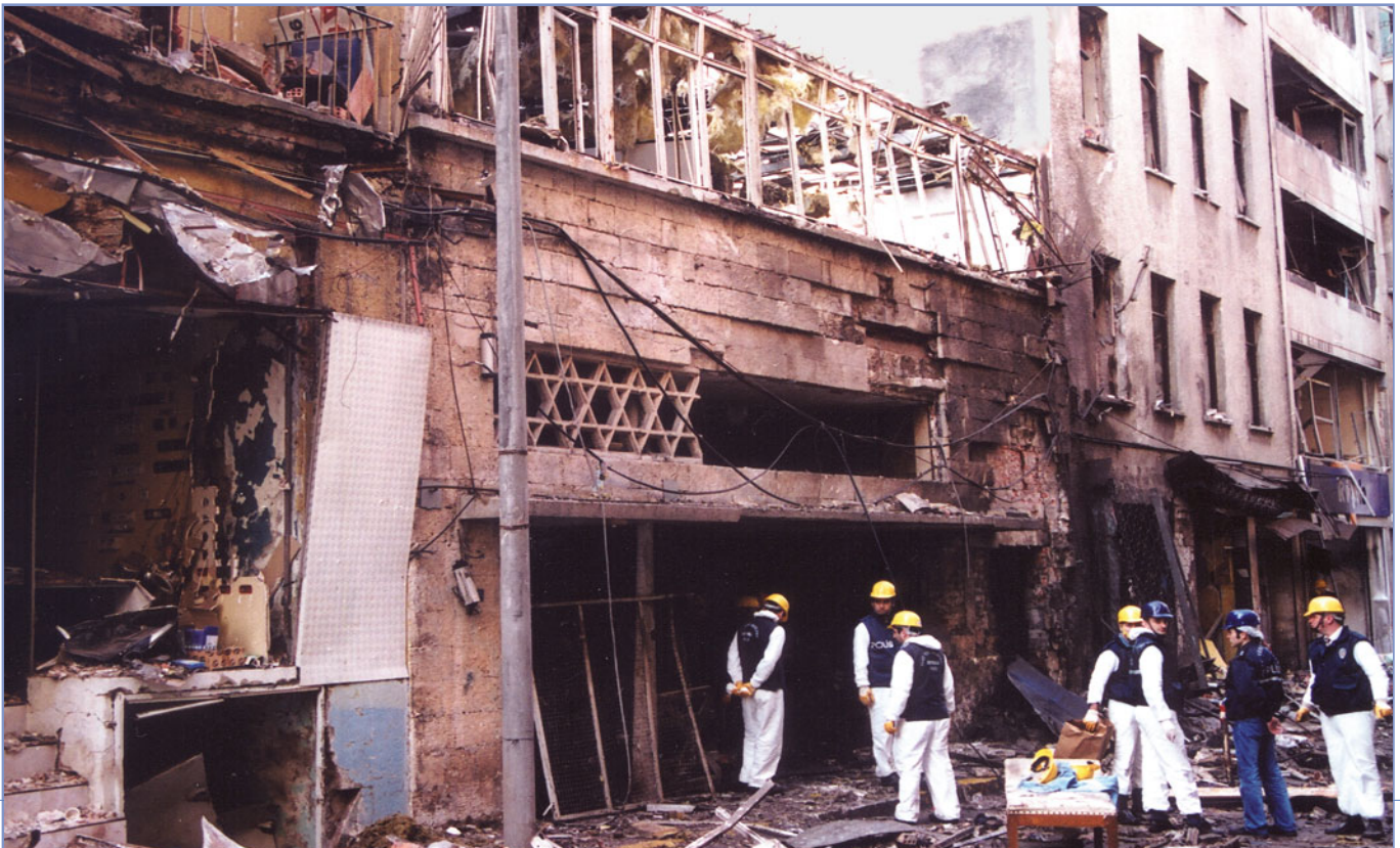
Bombed exterior of Neve Shalom Synagogue, Istanbul, Turkey, 15 November 2003
