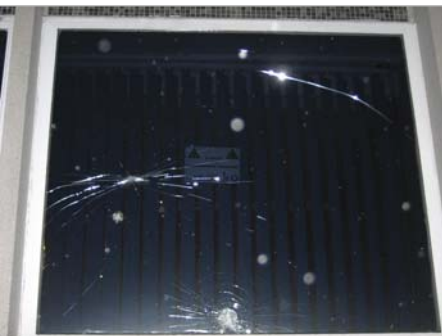
Arson attack at a London synagogue. CST's protective anti-shatter film on the windows prevented the arsonists from attacking the interior.
