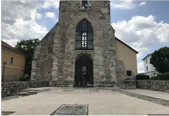
Figure 1. Tower of the Church of Mary Magdalene. Tower reconstructed, Nave — destroyed in the Second World War — foundations and walls marked.
